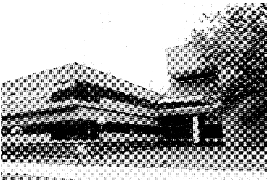
The new executive education building and Kresge Business Administration Library.
